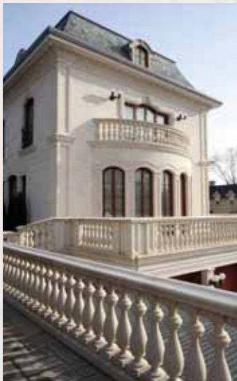
Architectural balustrades, columns, balusters, moldings and other architectural details are manufactured with the RIM process.
